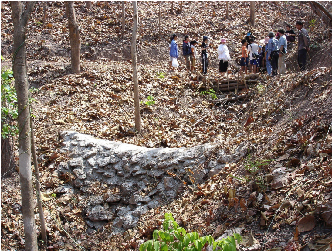
Figure 6. Two check dams in the mountains of Ban Samkha. Lower dam is made of cement and rocks. Upper dam (with children standing over it) is made of wood and leaves (photo credit: Arnan Sipitakiat).
